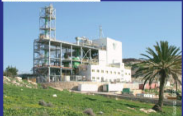
Demo Plant in Yblin, Israel
