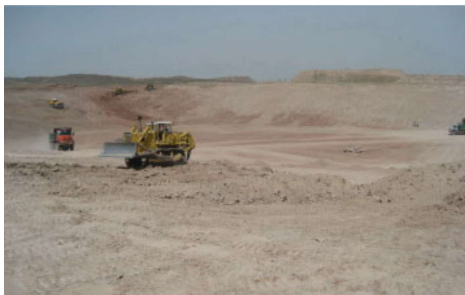
Figure 2: Tehran's new landfill
