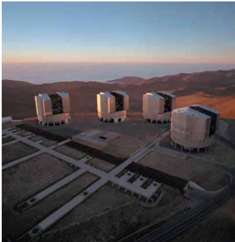
Figure 14 ESO's Very Large Telescope (VLT) array on the Paranal mountain in Chile consists of four 8.5 m diameter mirror telescopes. These telescopes can be coherently combined together with auxiliary telescopes (not on the picture but the rails are visible) to provide an interferometer with a baseline of up to 200 m).
