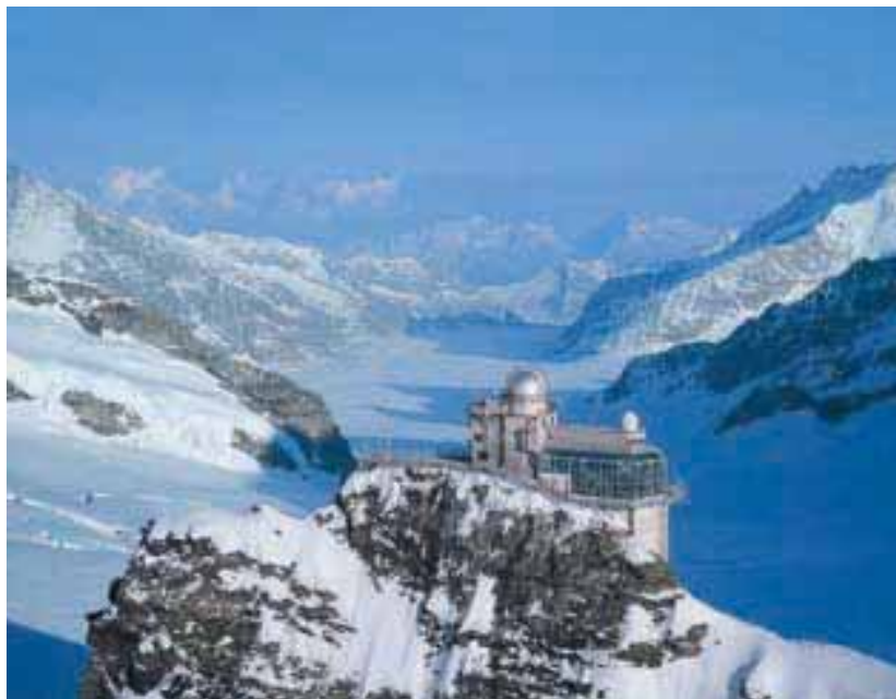
Figure 7 Two neutron monitors are installed at the Sphinx laboratory of the Jungfraujoch at an altitude of 3570 m. The 18-IGY-Detector is in continuous operation since 1958, while the Standard 3-NM64-neutron monitor operates since 1986.
