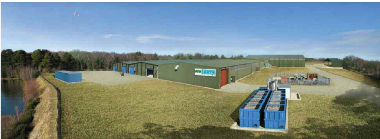
Fig. 16 Wimborne treatment facility
