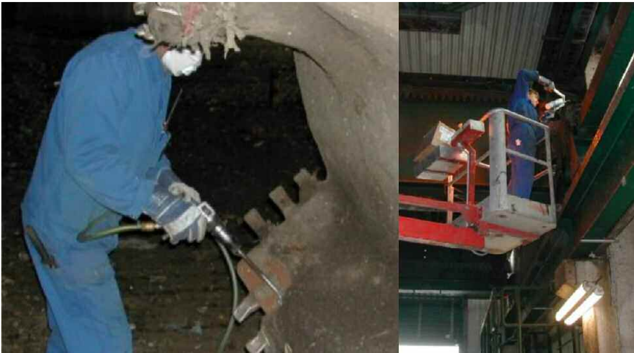
Fig. 4 Example: Maintenance of the equipment
