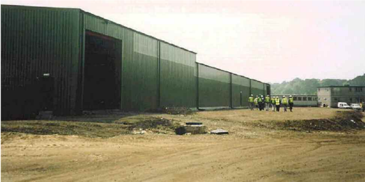
Fig. 1 Treatment facility in Wimborne
