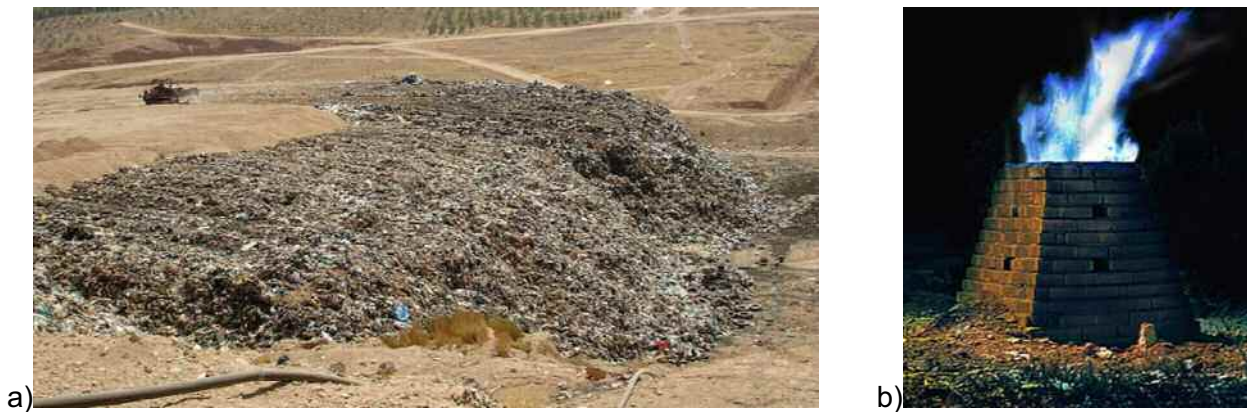
Figure 4 Shiraz Landfill: a) Daily covering and gas collection pipes; b) Biogas burning wells
