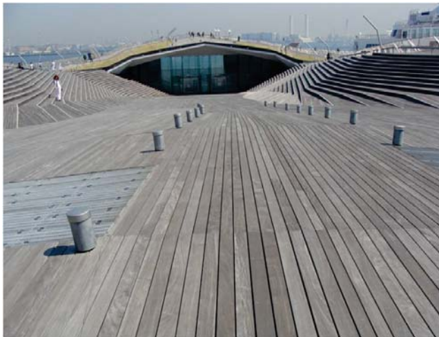
Abb. 5: Kreuzfahrtterminal Epe Deck, Yokohama
