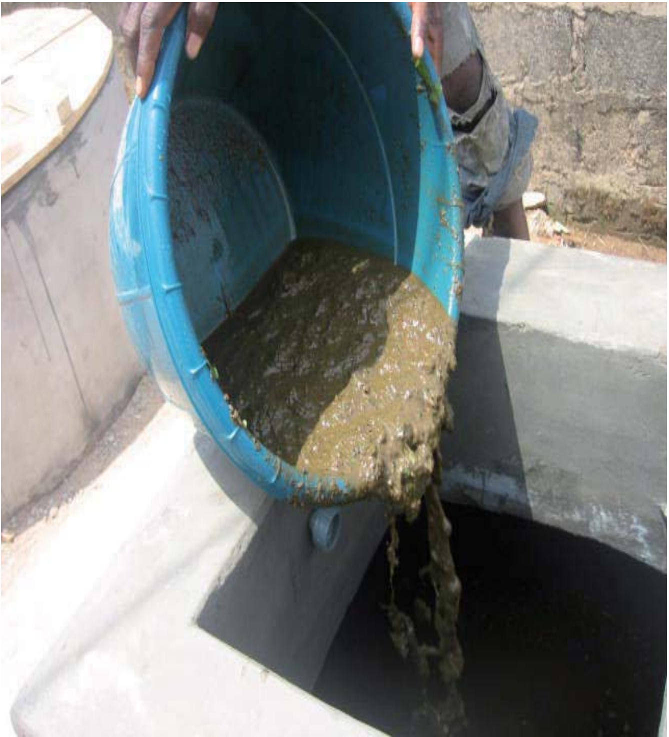
Fig. 5: The Charging of the Digester
