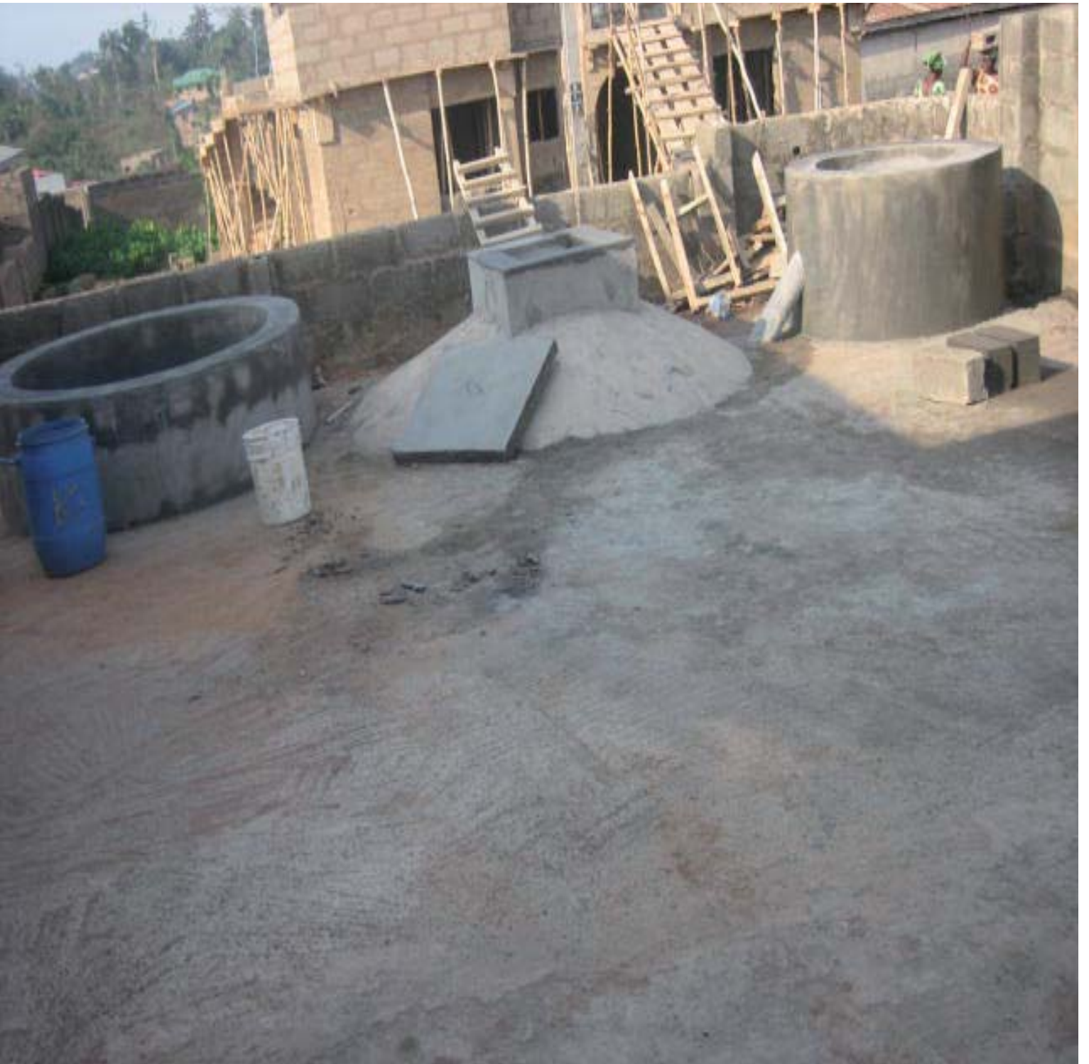
Fig. 3: The underground bio-digester made of concrete with inlet and outlet tank.
