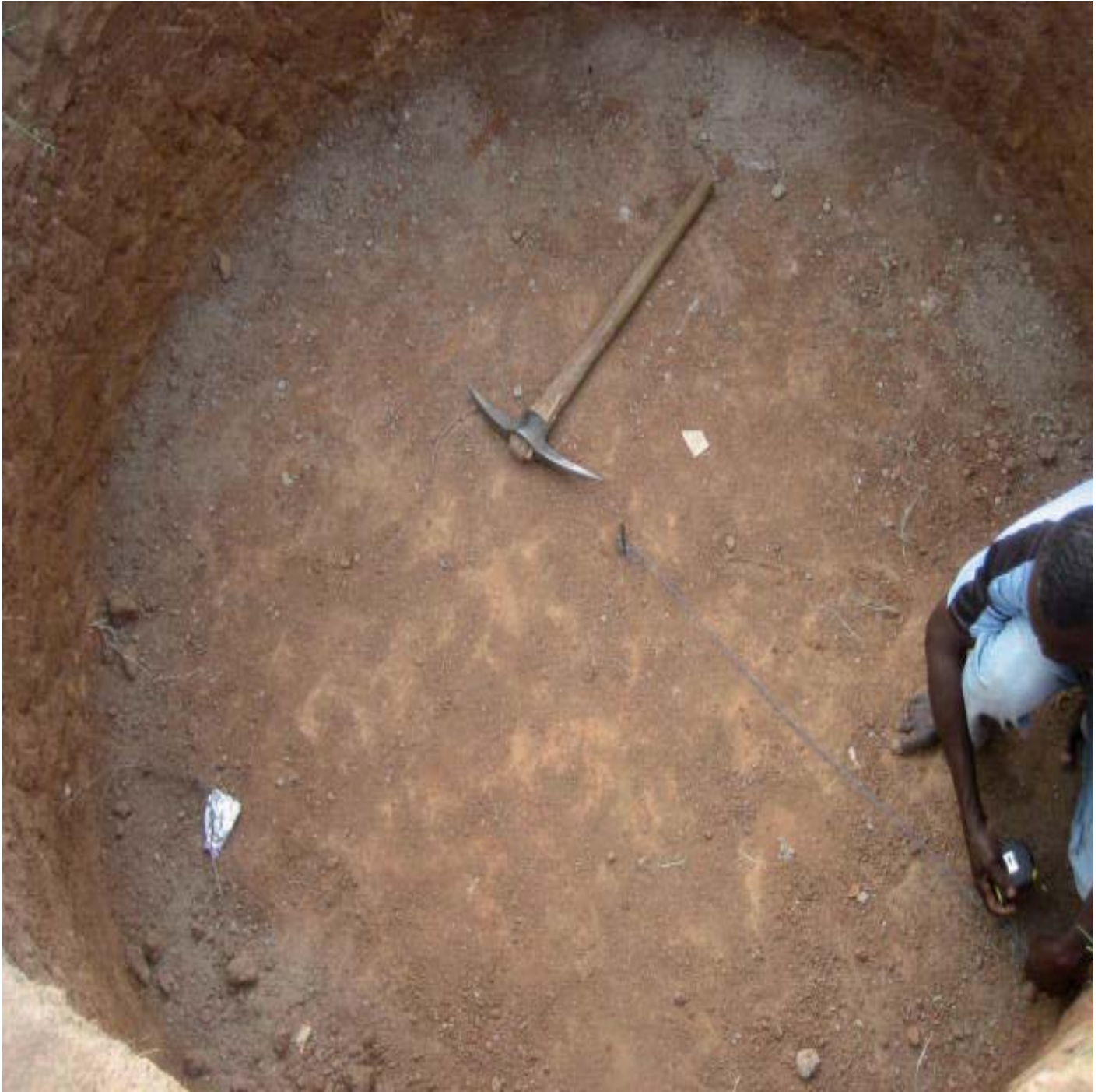
Fig. 1: The digging of the Digester
