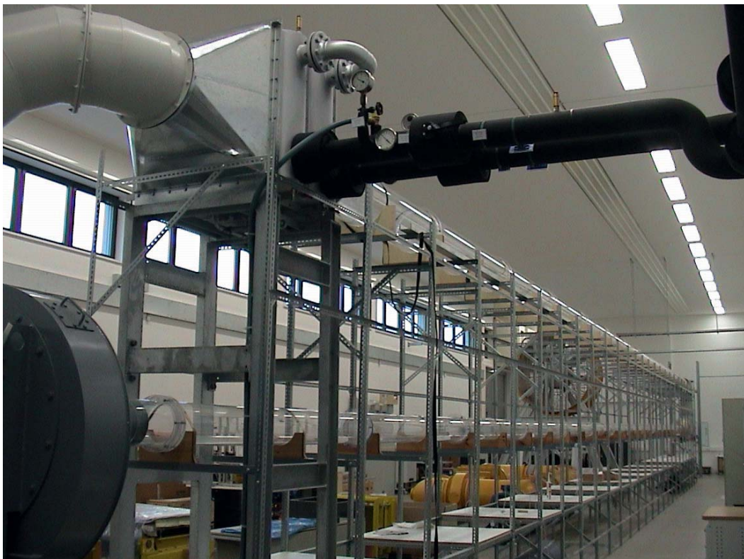
Figure 4.13: Rear view of the test facility from the blower and cooling unit with the actual test section and the return line.
