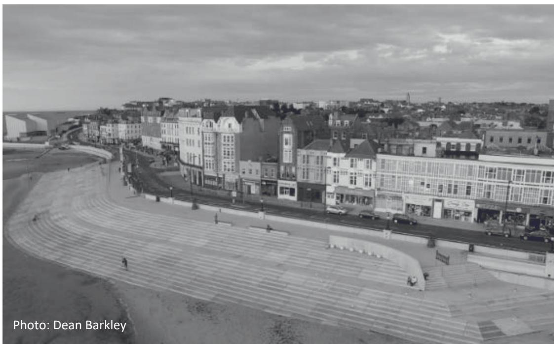
Figure 1: Stepped revetment at Margate, United Kingdom
