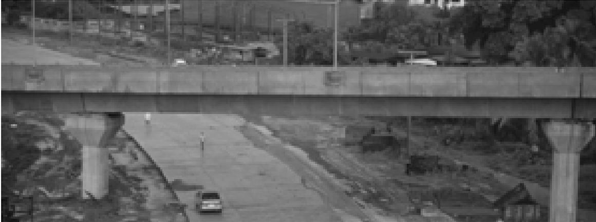
**Figure 1.7** Standard span  $l = 43.25$  m of the Second Stage Expressway (SES)
