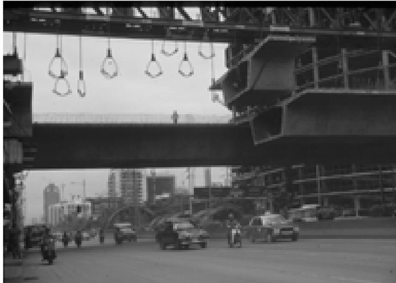
**Figure 1.6** Segmental bridge constructions in Bangkok
