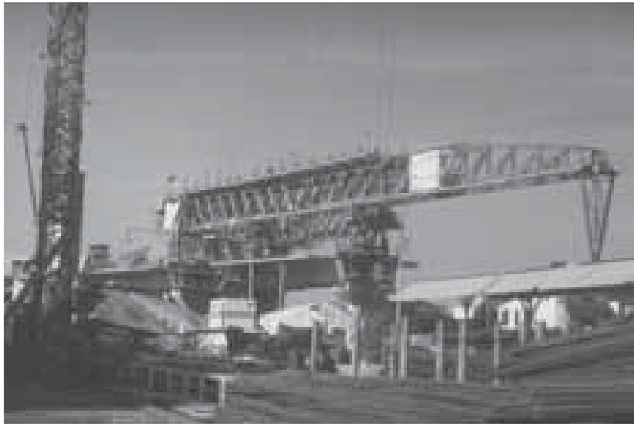
**Figure 1.5** Span by span method of construction (overslung truss)
