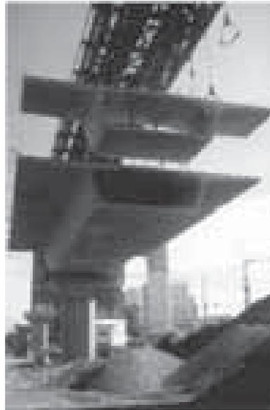
**Figure 1.2** Segmental hollow box girder bridge (SES Bangkok)
