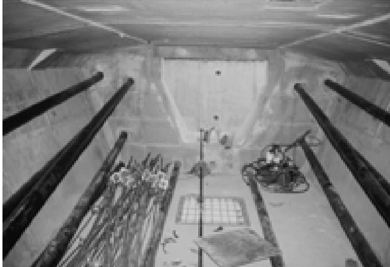
**Figure 1.3** Externally prestressed segmental bridge (SES Bangkok)–pier segment
