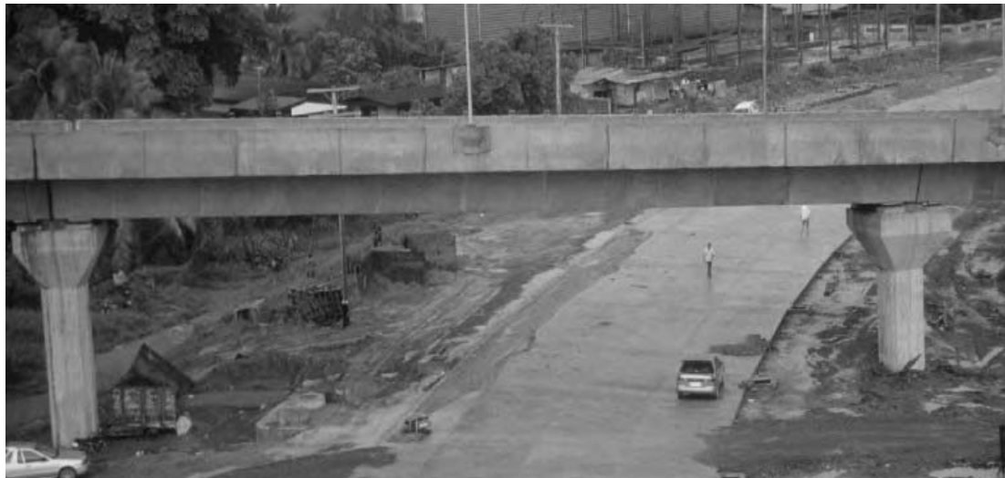
Figure 4.1 Span of the Second Stage Expressway segmental bridge in Bangkok [Ro1]
