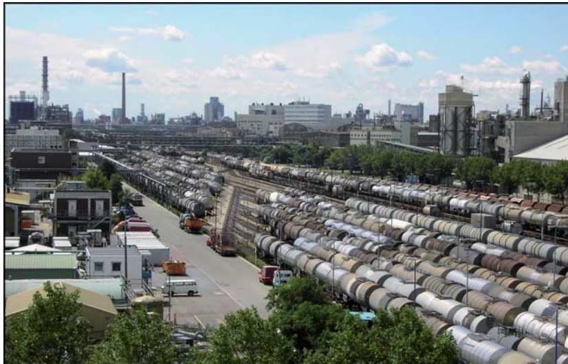
Figure 1.3. One of the rail yards at the site of our practical partner: BASF, The Chemical Company, Ludwigshafen
