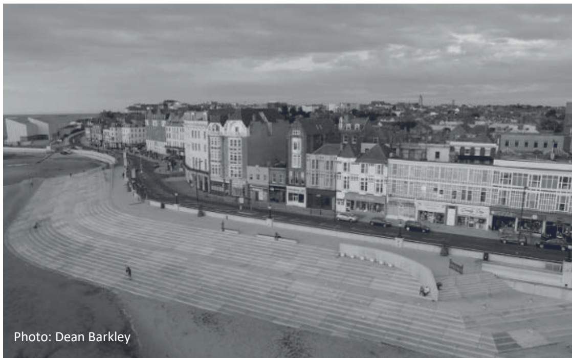
Figure 1: Stepped revetment at Margate, United Kingdom
