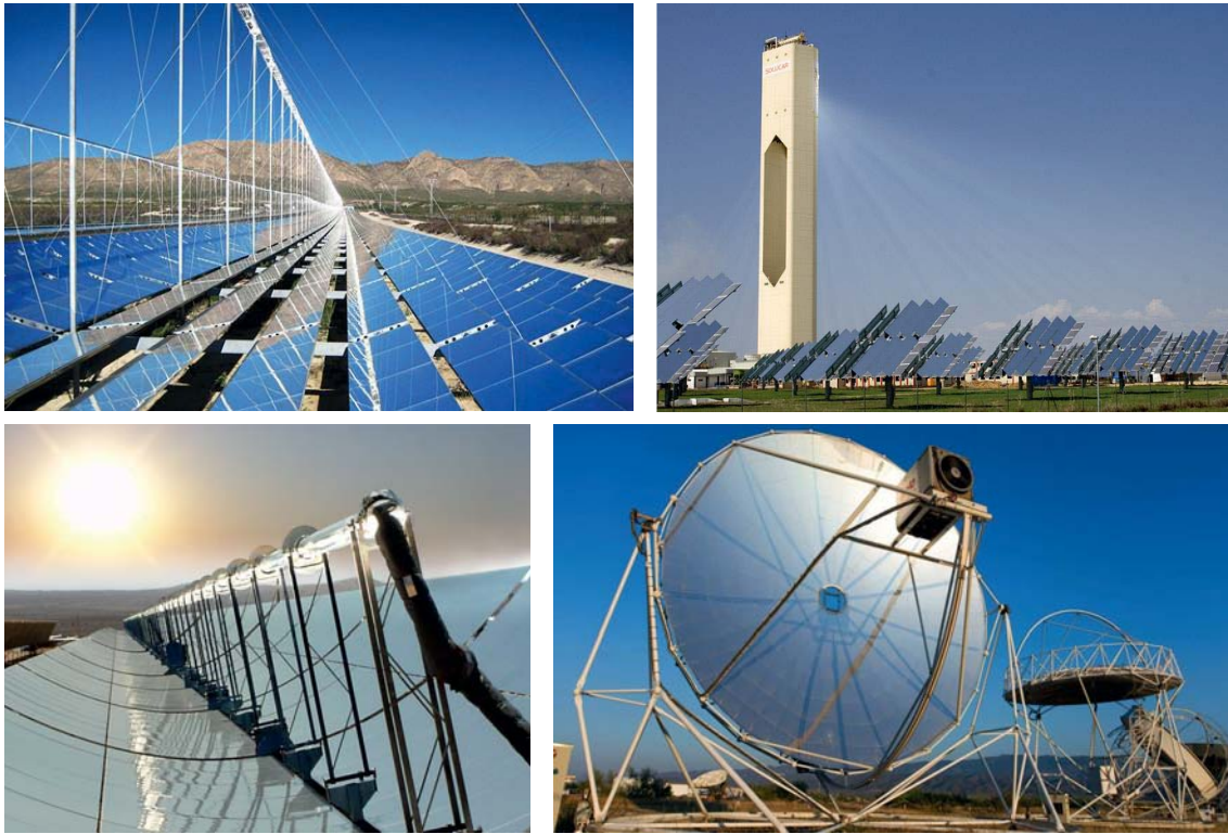
Figure 1.1: Overview of different CSP systems. Upper left: linear Fresnel collector (© DLR/Novatec), upper right: solar tower (© NARED/Abengoa), lower left: parabolic trough (© Schott AG), lower right: parabolic dish (© DLR).
