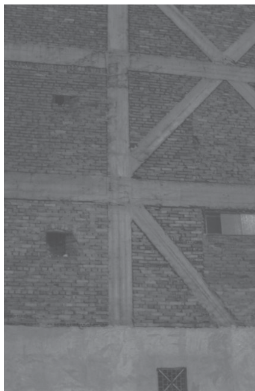
Figure 4.8: Detail view of reinforced concrete diagonal braces within a reinforced concrete frame structure for a building in Bucharest
