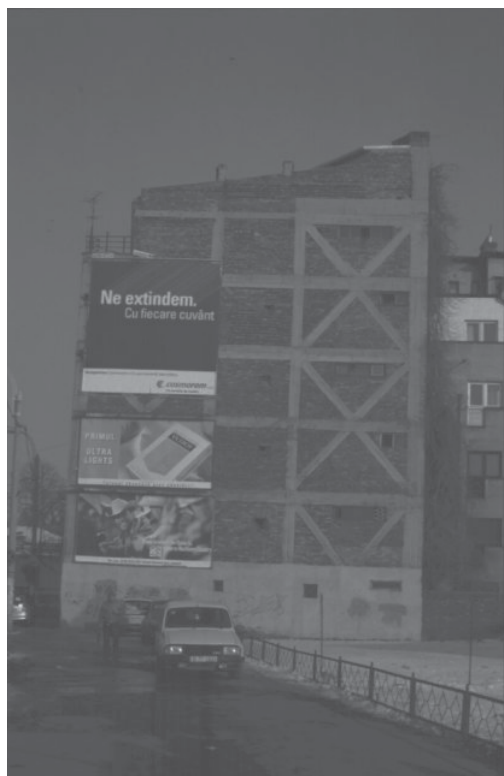
Figure 4.7: View of a building in Bucharest with reinforced concrete frame structure and diagonal braces
