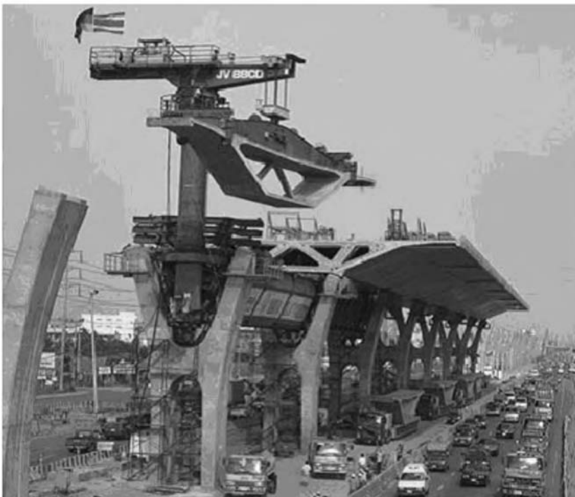
Figure 1.1 Segmental bridge construction in Bangkok [Br5]
