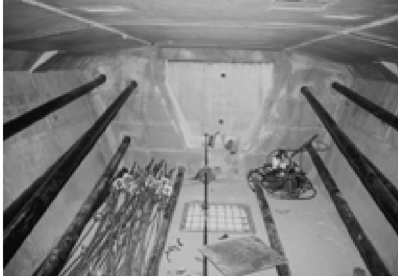
Figure 1.3 Externally prestressed segmental bridge (SES Bangkok)–pier segment
