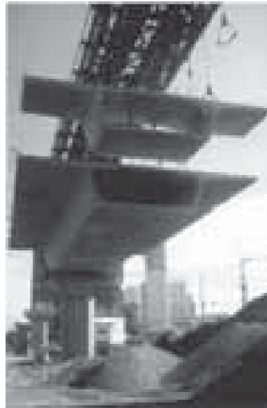
Figure 1.2 Segmental hollow box girder bridge (SES Bangkok)
