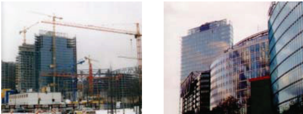
Figure 1: Images of the Potsdamer Platz in Berlin: The left image shows the construction site of the Potsdamer Platz in 1998, when it was Europe's biggest construction site, while the right image shows the Potsdamer Platz now, in 2003.
